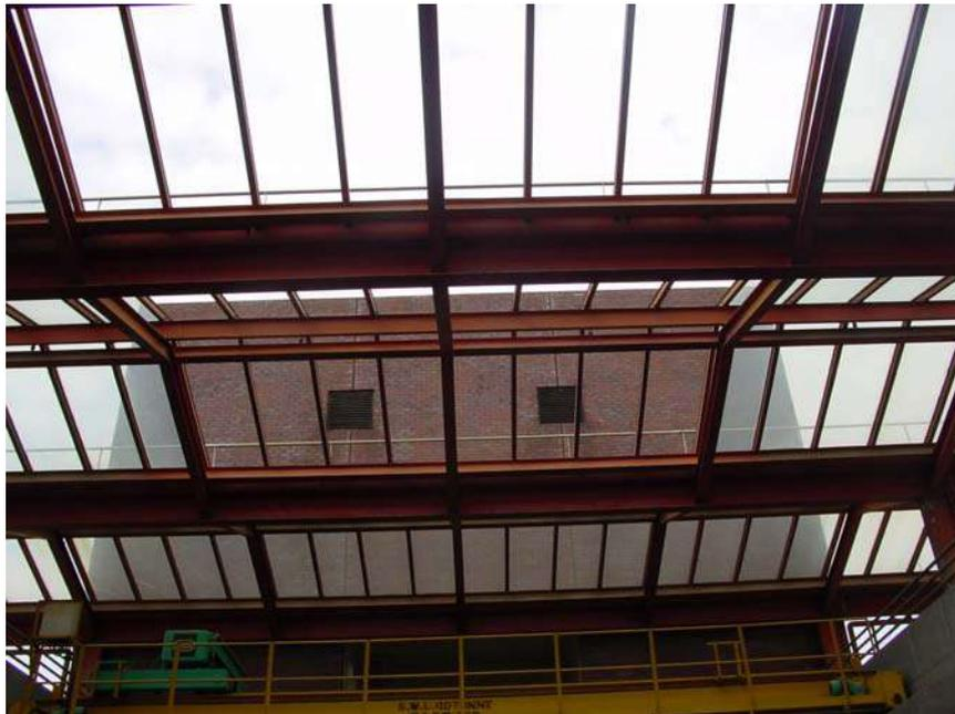
Damaged wired glass in center bays
