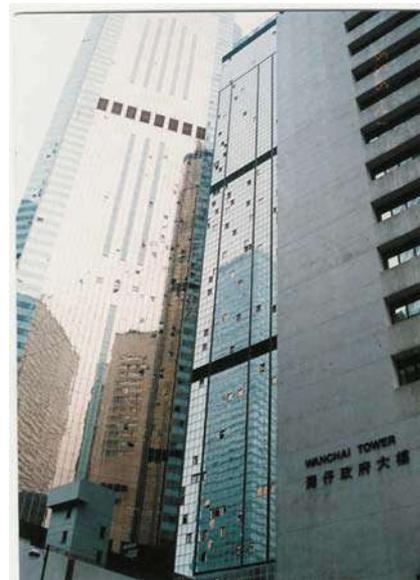
Damage of glass panels during typhoon
