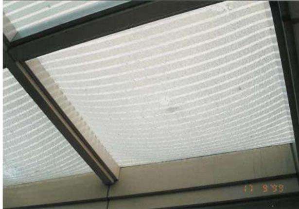
Damaged laminated glass panels at a cover walkway
